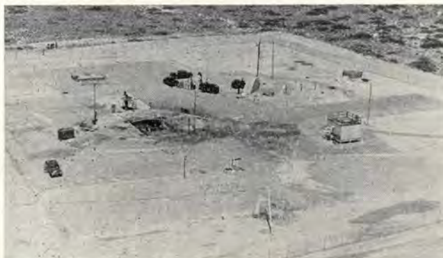
The silo cap doors lay 99 and 109 feet to the east and west.
